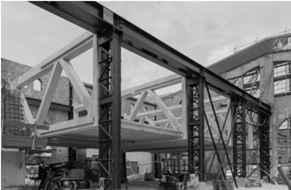
Gjuteriet transformation under construction. The new timber frame being rapidly assembled on site during summer of 2021.
